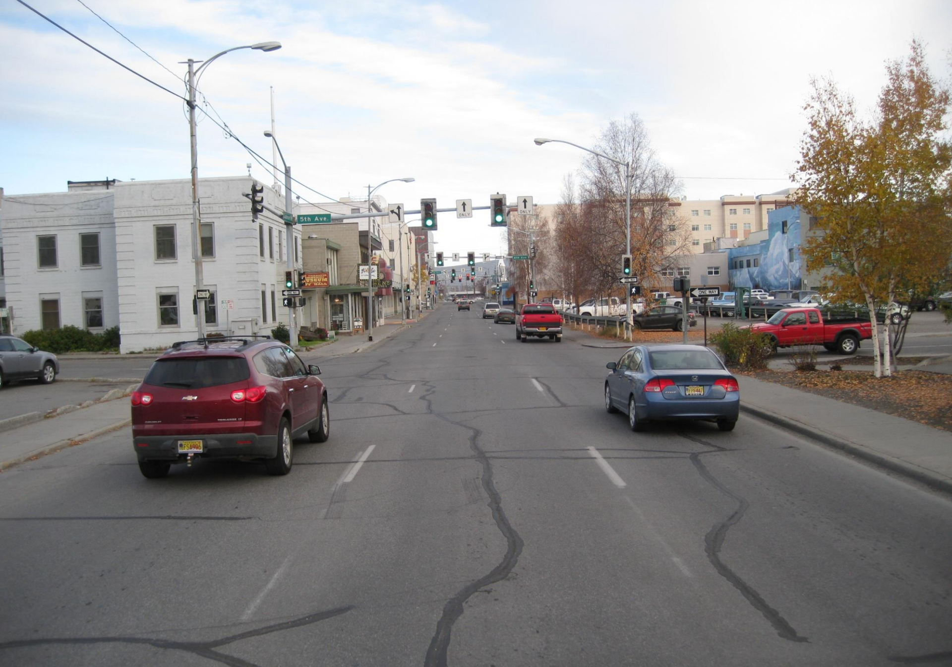
Cushman Street – Existing Condition (3 lanes)
