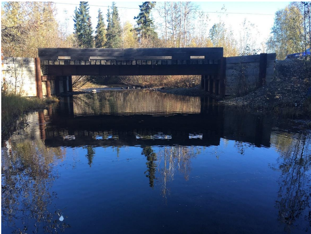
Site 4 September 10 th From center of channel looking downstream (north)
