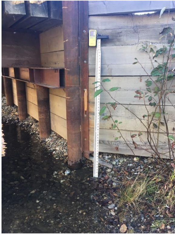
Site 4 September 10 th Benchmark on bridge right (east) abutment, upstream side
